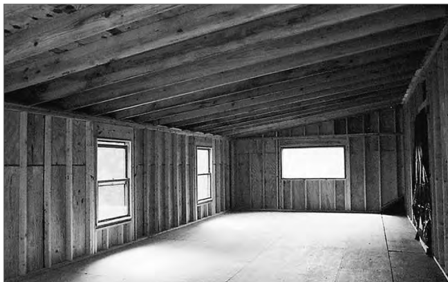
Expansion of office space at JPI during the first phase of construction. Photos © Patricia Smith
