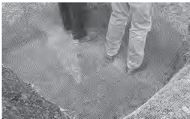
The pit is lined with a wire mesh.
