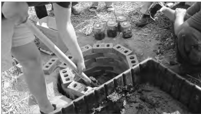
Putting the stirred manure into the brick pit built during the workshop and adding the compost preparations
