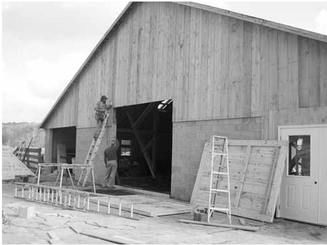
Work proceeds on the build-out of our barn
