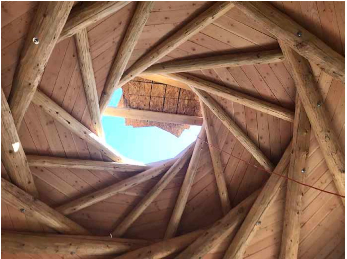
Spiral design roof structure
