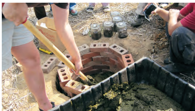
Filling pit with barrel compost
